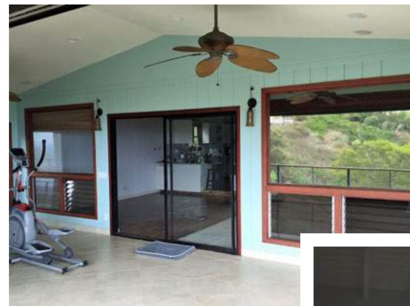
Before photo of enclosed lanai with the old kitchen in the far corner.
