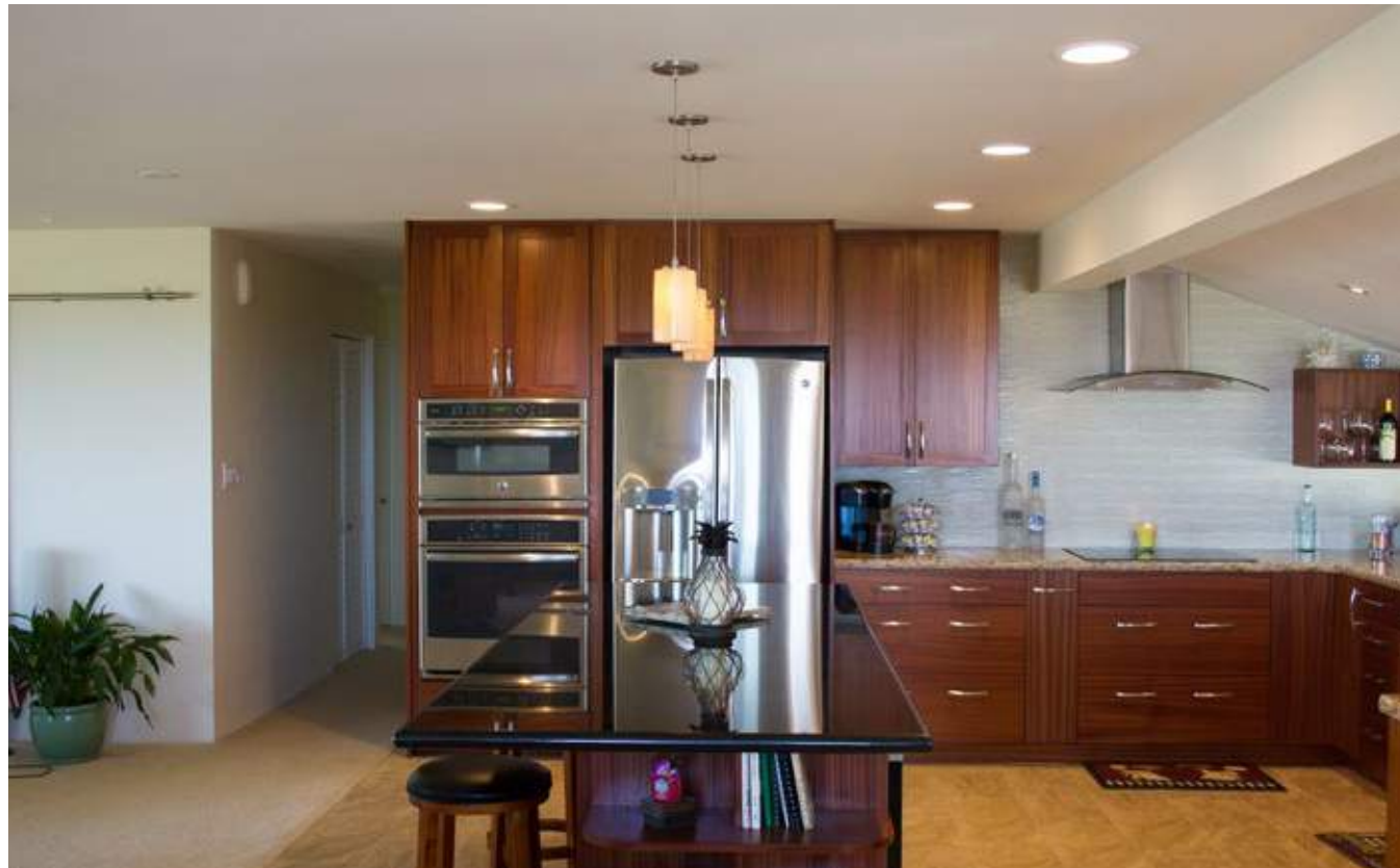
A ceiling beam replaced a load bearing wall taken down to enlarge the kitchen.
